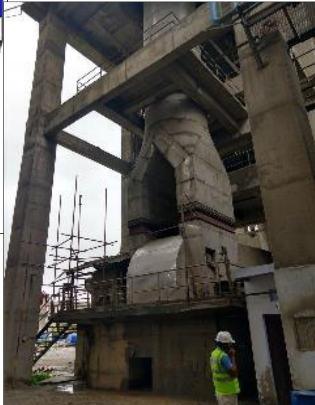
Existing Y piece cross section 3000 x 750mm
